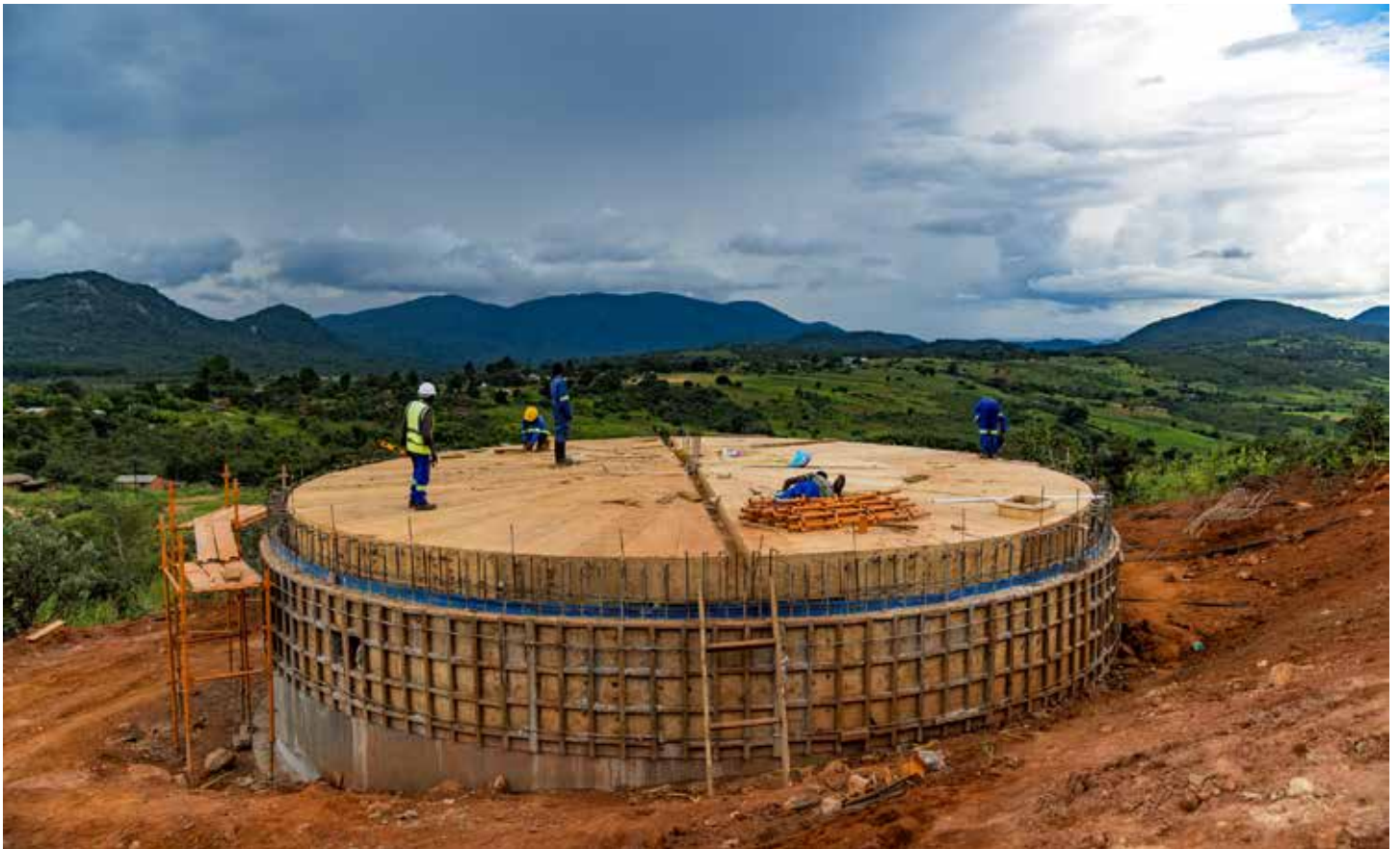
Work in progress at Nyika Vwaza treatment site.
