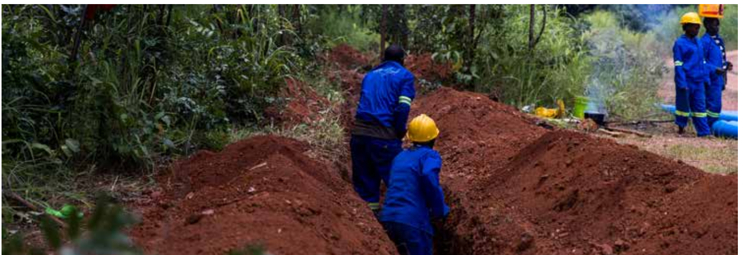
Work in progress – excavation of trenches for pipes.
